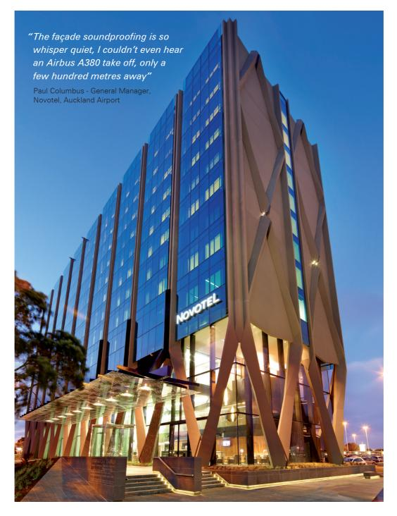
$\label{eq:Total clad solution} Total clad solution \\ Twin skin for high performance acoustic rating \\ Very low design noise level of 30dB, (L_{Aeq}) achieved in all hotel rooms$
